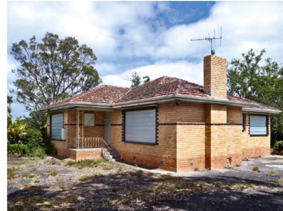
Triple Fronted Brick Veneer, Plenty Road, South Morang 2010, type C print edition: 6
